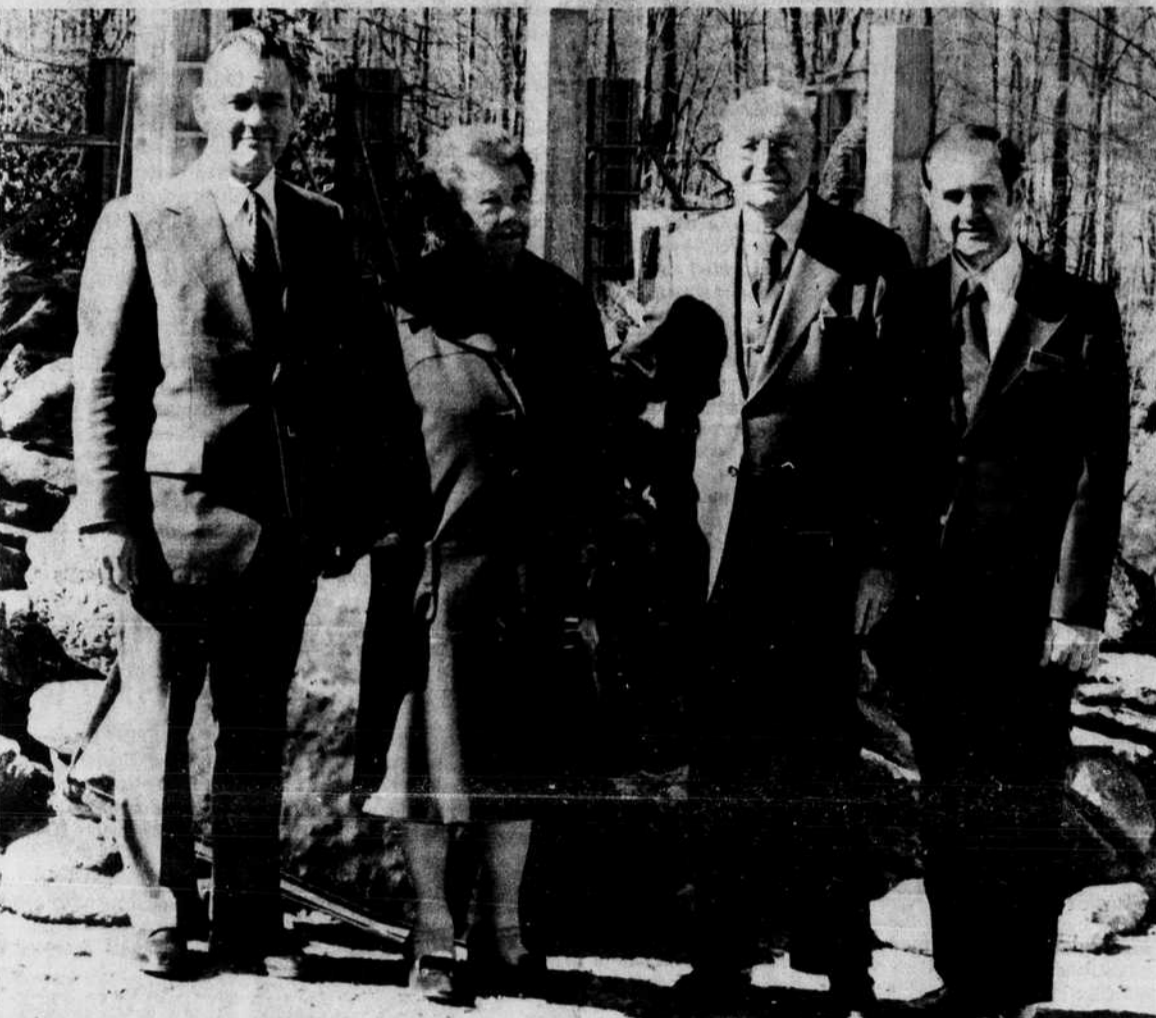
THE CONSTRUCTION in the background is for the new chapel at Blue Ridge Assembly. It will be a memorial to Paul Douglas and Ella Camp and is being given by their daughter Mrs. Billie Camp
