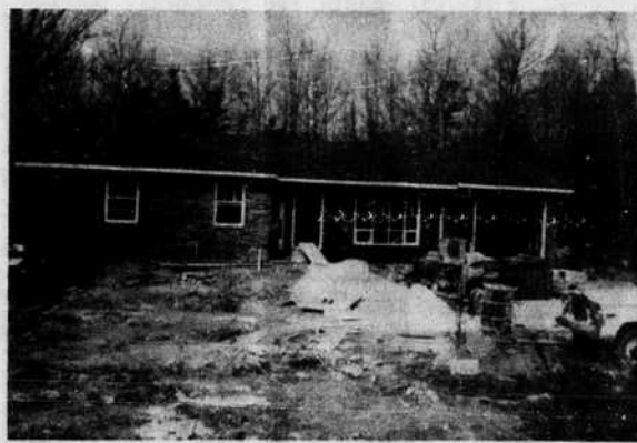
Under Construction - Home of Mr. and Mrs. Buford Copeland
