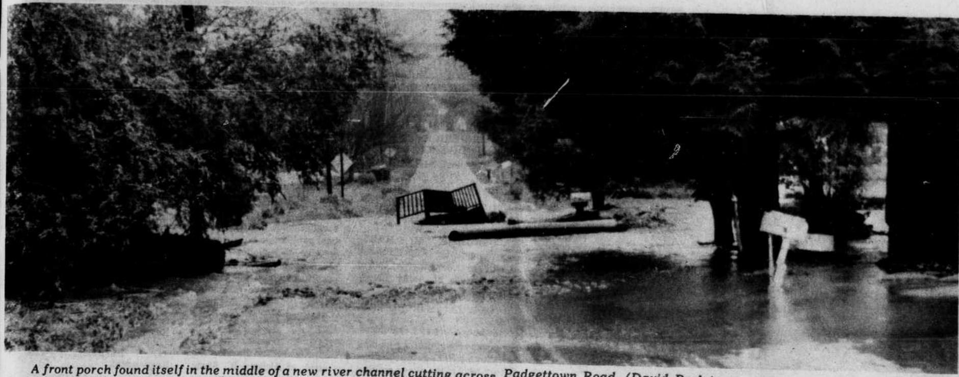
A front porch found itself in the middle of a new river channel cutting across Padgettown Road. (David Peele)
