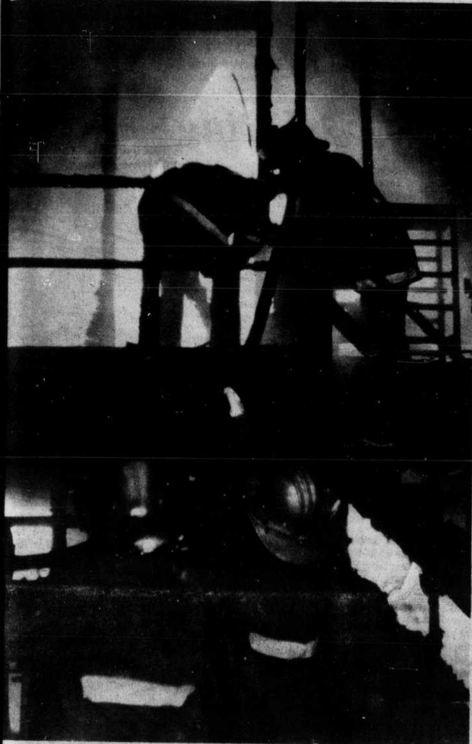
Black Mountain Firemen hand hose up a charred stairway to put out flames second level of A-frame at Travel-Eze Motel. (Dan Ward)
