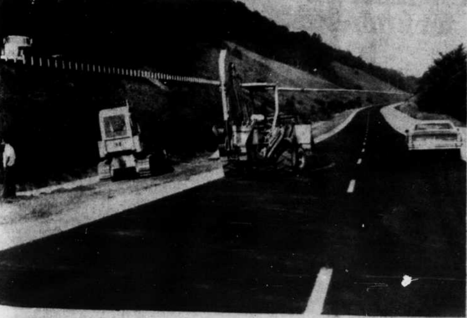
Cars and construction crews share the unopened portion of I-40. (Clint Williams)
