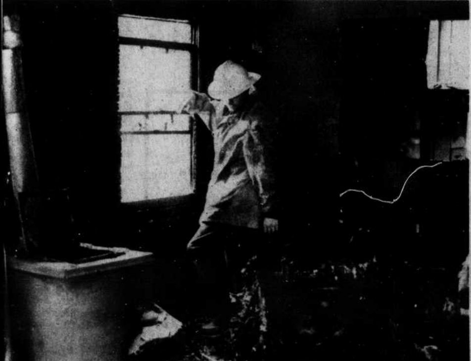
Assistant Black Mountain Fire Chief Sterling Poe inspects damage at scene of a house fire on Tabernacle Road. (Dan Ward)
