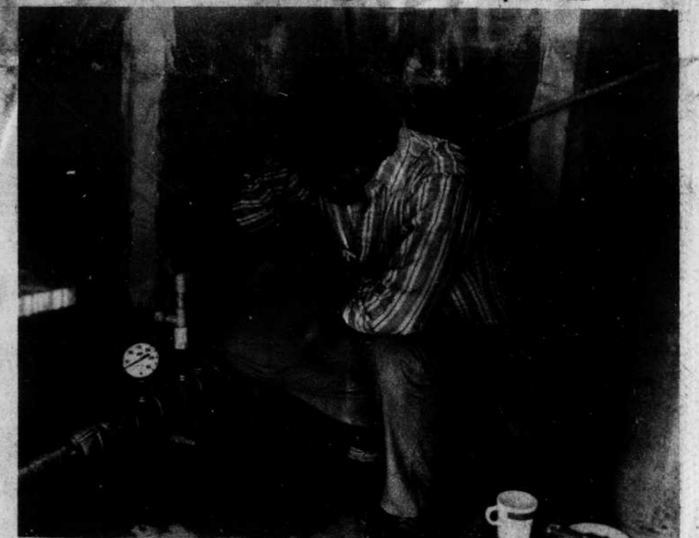
A Black Mountain employee checks the pressure on the new pump at the golf course. (Dan Ward)
