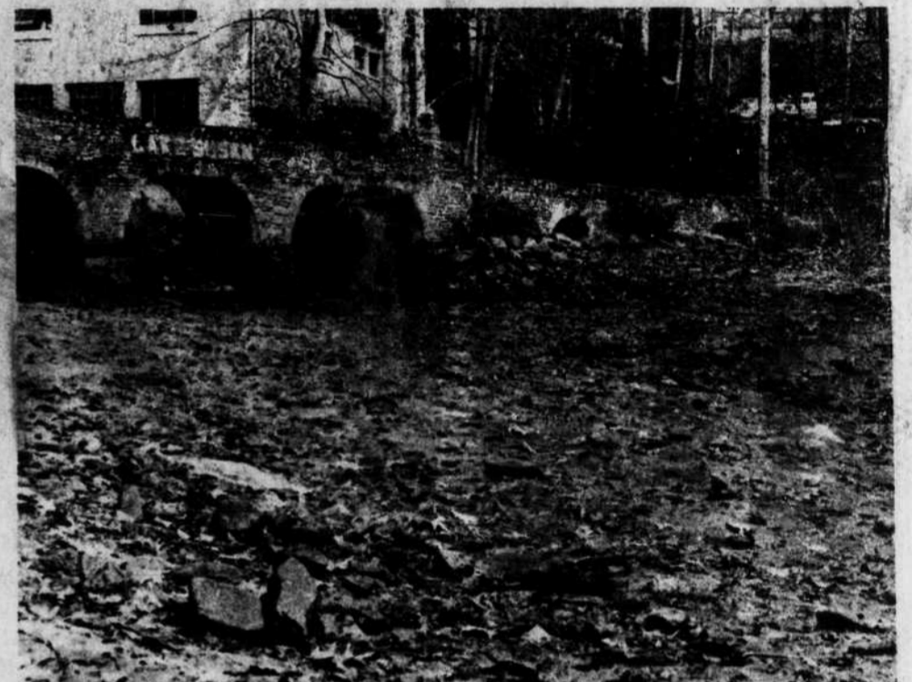
Lake Susan was once again a crater last week when it was drained to replace fill that had washed out at the base of the dam. The contractor who repaired the dam last year replaced dirt fill with clay at no cost to the Mountain Retreat Association. (Dan Ward)
