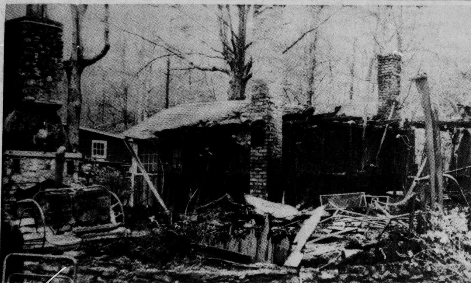
Chimneys and plumbing pipes stand as grim sentinels at the former home of Ridgecrest residents after a fire destroyed the structure early last Sunday morning.
