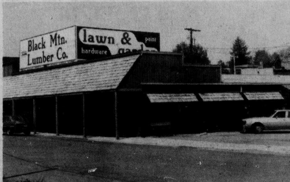
Black Mountain Lumber Company has completely renovated the facade of its main building by repainting and the addition of a shake covered roof over the sidewalk.
