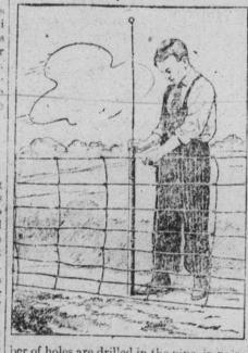
ber of holes are drilled in the pipe, in pairs at equal distances apart, and a small loop made of wire is inserted into each, The vire fonce is then stretched in the usual , and a long straight piece of heavy wire is slipped down through the small loops to hold the fence in place. With this rrangement the fence may be put up or
