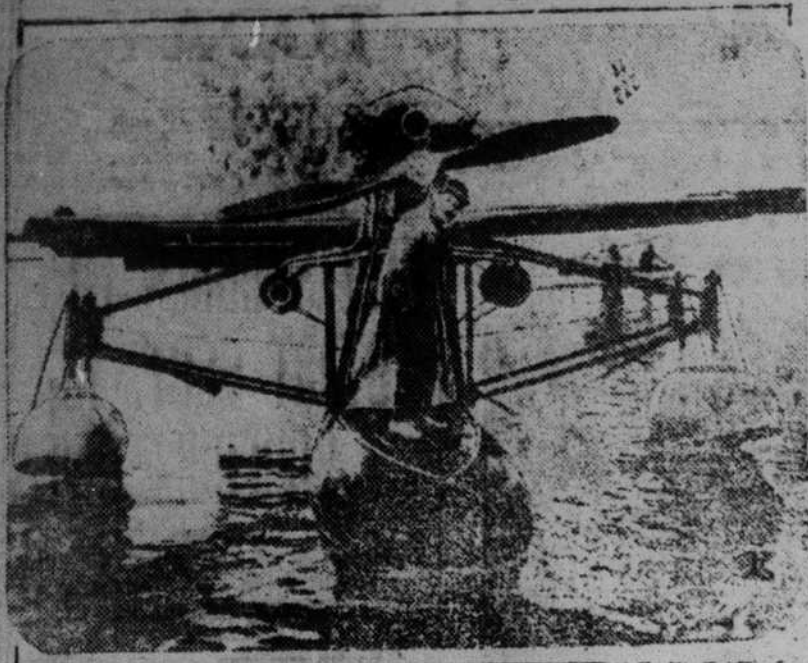
The "Sea Flea," an ingenious combination of ship and airplane, is shown here with its inventor, H. G. Bennett, a former engineer. The old craft is being tested near Jacksonville, in anticipation of the transatlantic flight attempt. Its average speed is 100 m.p.h., and it has a range of 150 miles in 2007.
