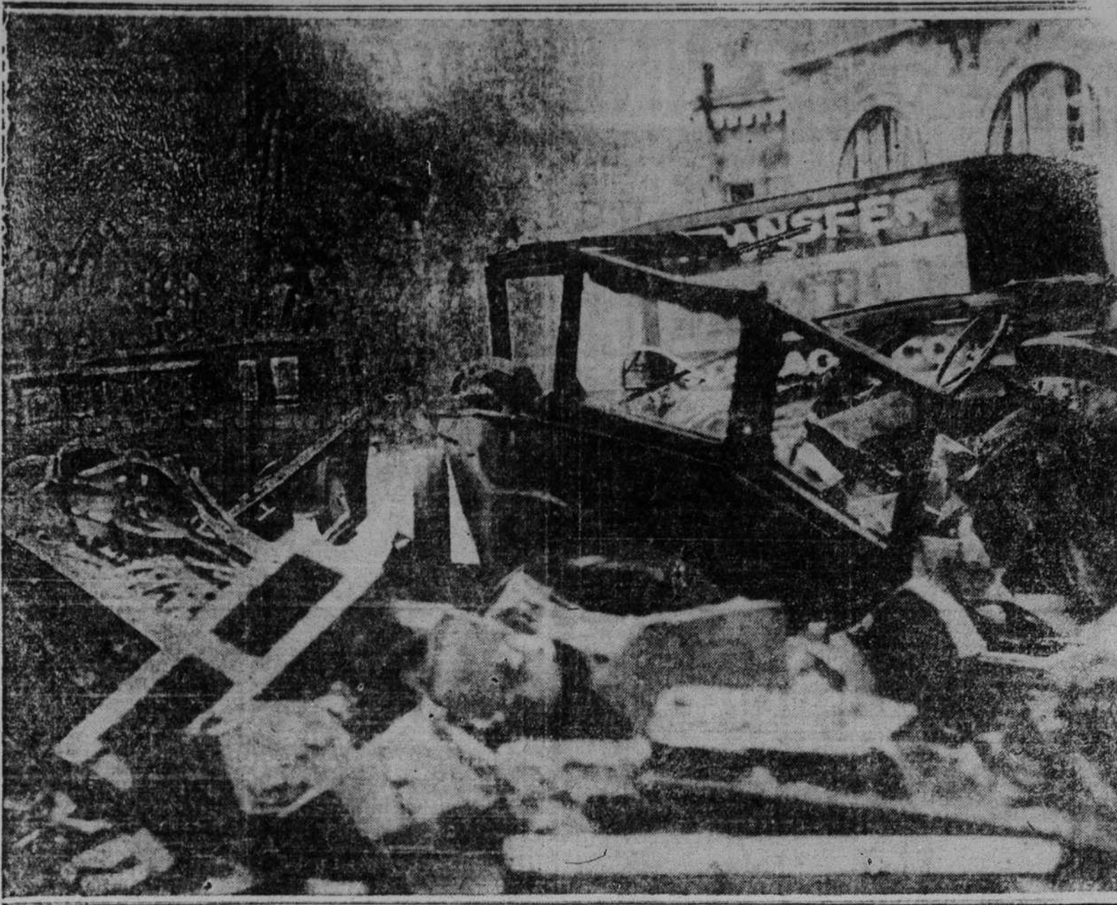
And rather badly used, too. The storm wreaked a terrific bit of damage here, piling up automobiles and trucks and smashing them with stones from buildings. In the
