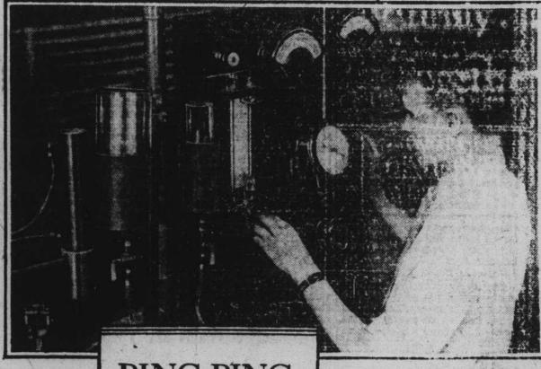
PING, PING, The anti-knock qualities of Esso are constantly being tested in the PING, spells "Standard" laboratories on "knock-testing" machines like that shown in this picture. This is one of the many precau-Lost Power tions taken to maintain in Esso the lowest of all knock ratings.
