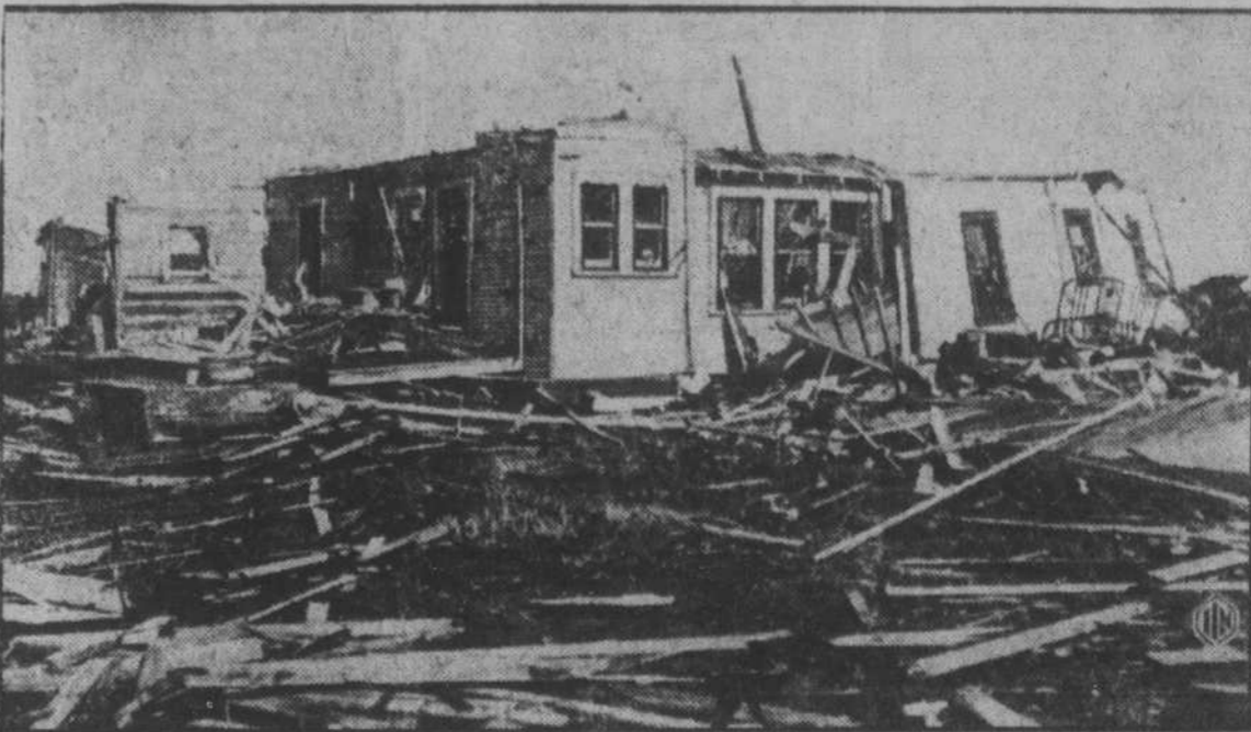
Wrecked by a disastrous tornado, this once cozy residence crumbled over the bodies of John Edwards, his wife and their two children. Twenty others are said to have had their lives snuffed out in the twister which struck Bethany, a suburb of Oklahoma City.
