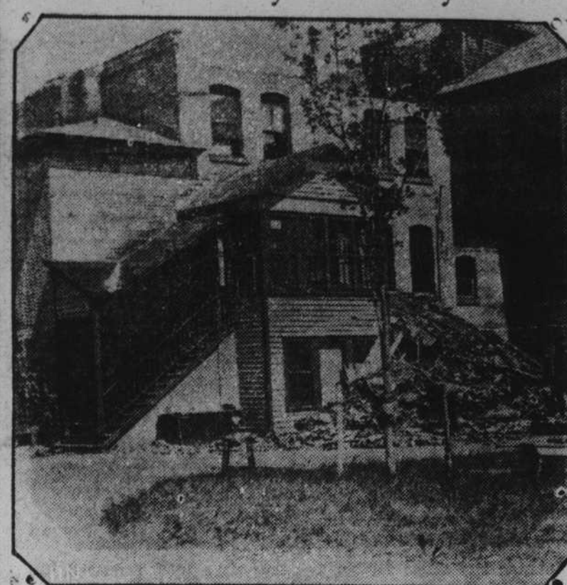
Investigation has been launched at Houghton, Mich., into the death of three inmates of the county infirmary who were killed when a 60-foot chimney crashed through the roof of the institution during a severe wind and rain storm. Ten inmates were buried in the debris.
