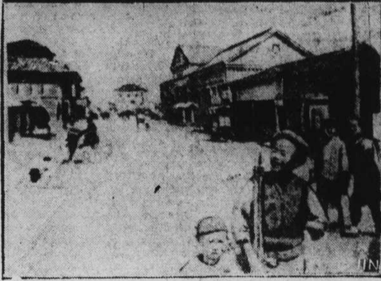
Railway station and thoro fare in Taikoku, capital of the Jap- anese island of Formosa where more than 3,000 were killed by an earthquake.
