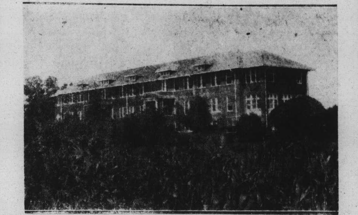
This township institution now has 70 beds. The addition made possible by donations from A. H. Webb, A. C. Miller and Duke Foundation has been completed and was dedicated Monday. The addition and equipment cost $37,000. The maternity section on the second floor is a memorial of the late Mrs. Eliza Webb.
