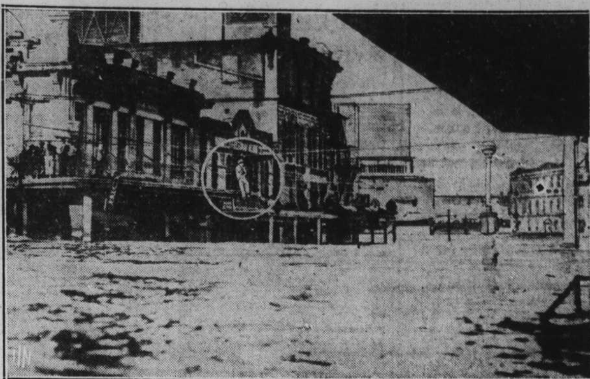
A breeches buoy is utilized to rescue men marooned in the building at the left as flood waters from the Buffalo Bayou inundated Houston, Texas. Seven were drowned and the property damage was estimated at $2,000,000 as the flood waters receded.
