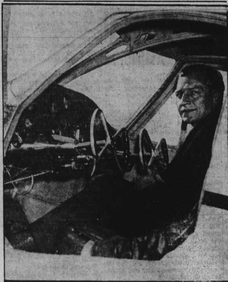
U. S. TESTS FLIVVER PLANES —Eugene L. Vidal, director of the bureau of air commerce, "lands" the second of the government's low cost "foolproof" flivver planes in Washington. The government contemplates purchasing six of the light ships if they pass final tests. The flivver plane has a wing spread of 35 feet and an overall length of 25 feet 6 1/2 inches.
