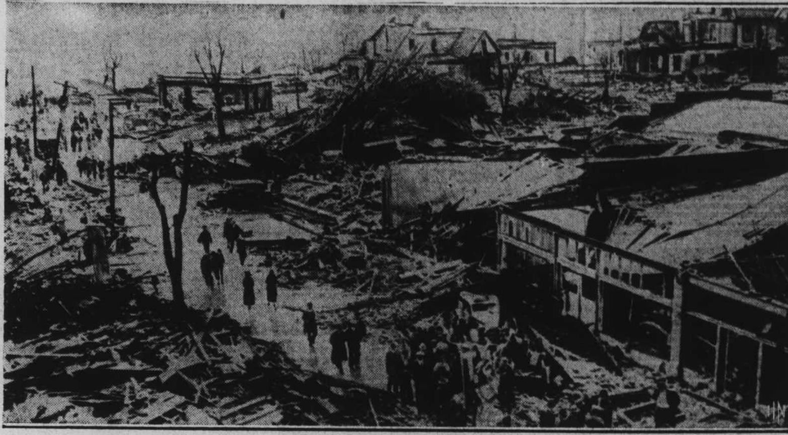
Frame and brick buildings alike were blown to the ground at Gainesville, Ga., as this photo of the city's square dramatically shows. Terrific rains have swollen rivers in the seven southern tornado-torn states and floods threaten to add to the destruction of the wind.
