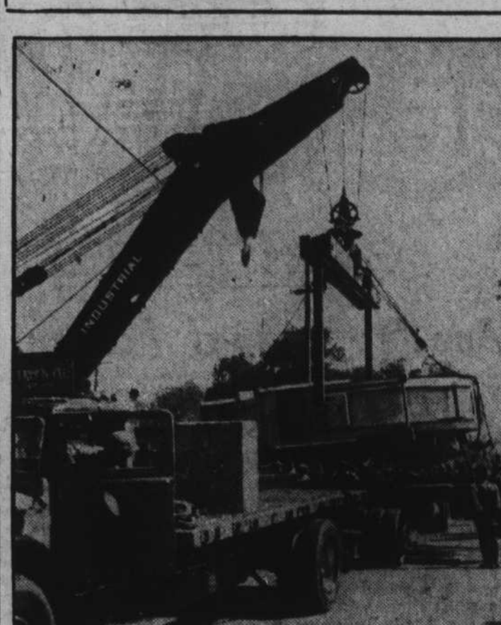
Workers required just seven hours to transfer this $2,000,000 piece of glass from railroad car to truck after its arrival at California Institute of Technology, Pasadena. During the next four years, the glass will be ground into a mirror for the 300-inch world's largest telescope, atop Mt. Palomar. The telescope, with the new mirror, will extend vision twice as far as any other.
