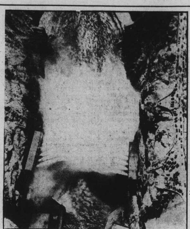
Here is the scene from the air as 3,600,000 cubic feet of water rushes from 12 Boulder Dam outlets each minute, generating electric power for western cities. The giant federal project was put into full operation when President Roosevelt pressed a button in Washington, D. C., on the opposite side of the continent.
