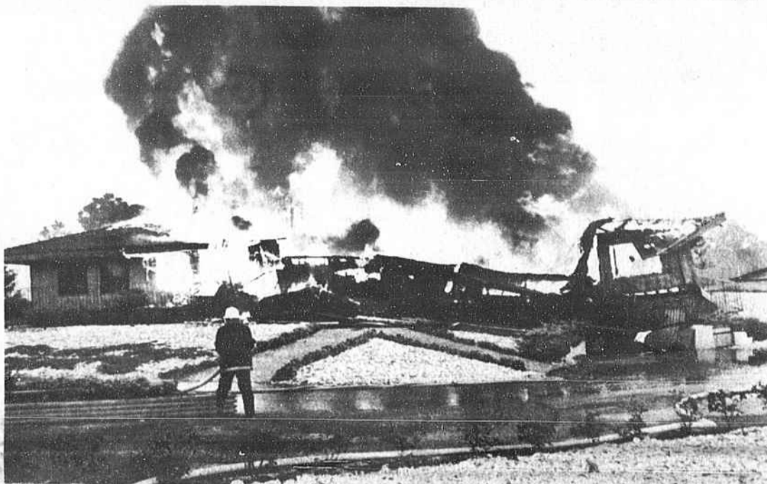
VOLUNTEER FIREFIGHTERS and rescue workers from Calabash to Supply responded when fire broke out Friday night in a golf cart storage area of the Oyster Bay clubhouse. Despite their containment efforts, the blazed leveled the structure.
