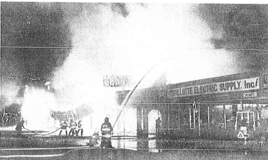
A NEW DOUBLE FIRE WALL stopped the fire at Shallotte Electric Supply, which reopened for business almost as usual Tuesday with some smoke and water damage. The seven remaining stores were razed, including four occupied by businesses.
