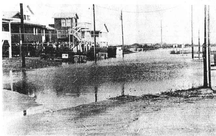
STAFF PHOTO BY SUSAN USHER WITH ITS BROAD STRAND and deep frontal dunes, Sunset Beach sustained less oceanfront structural damage than other areas. However, 25 to 30 feet of fron-
