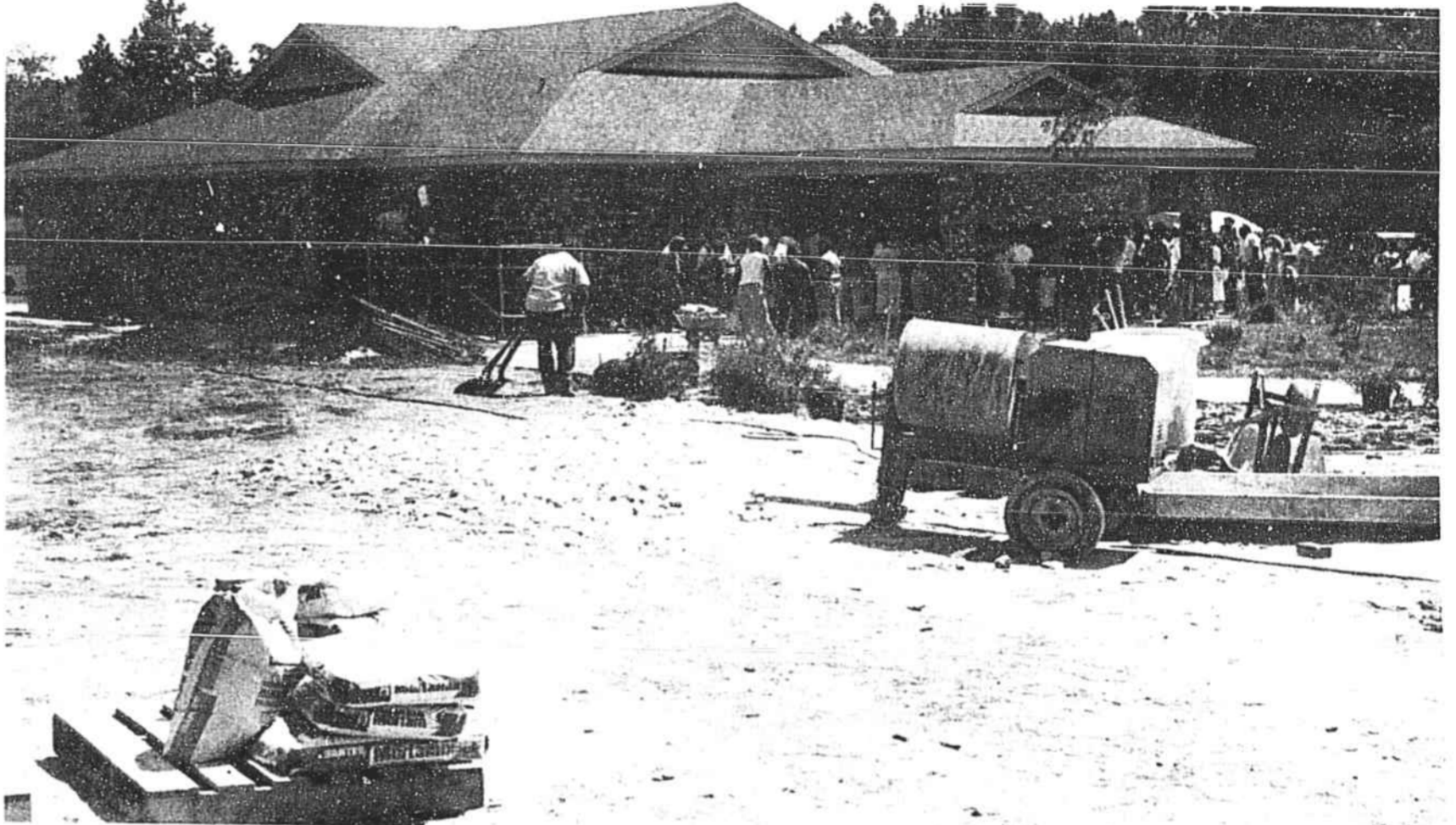
A FEW BAGS of dried cement and scraps of wood were all that remained on the ground when the building was completed about 3 p.m. Sunday. In this
