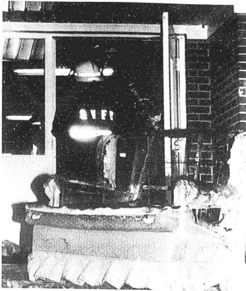
DAMAGE from a fire at Brunswick Village Residential Care Facility in Shallotte last Wednesday afternoon was limited to the west wing room where the fire began in this chair, which firefighters set outside.
