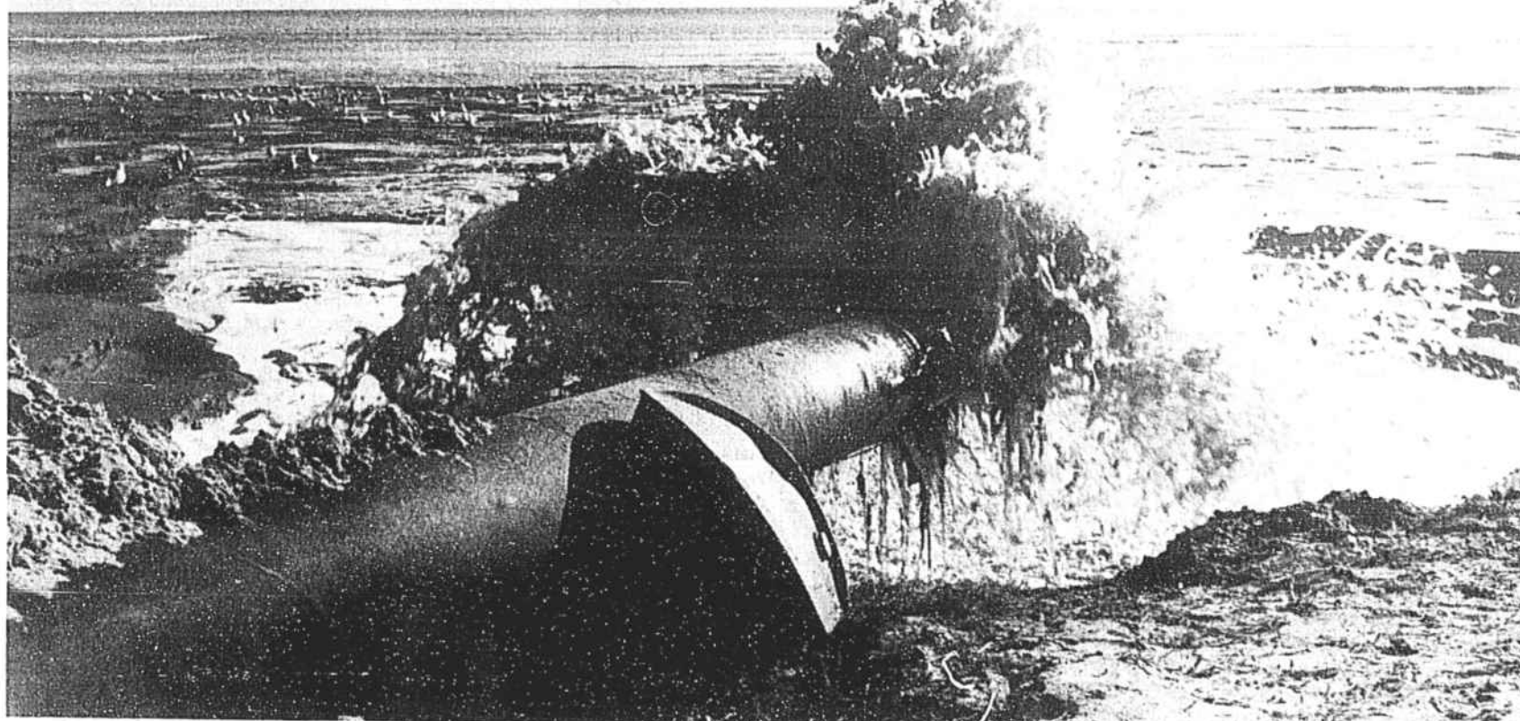
SANDY SPOIL flowing from this pipeline is expected to help rebuild the erosion-battered east end of Holden Beach. A dredge boat is pumping the sand from Lockwood Folly Inlet.
