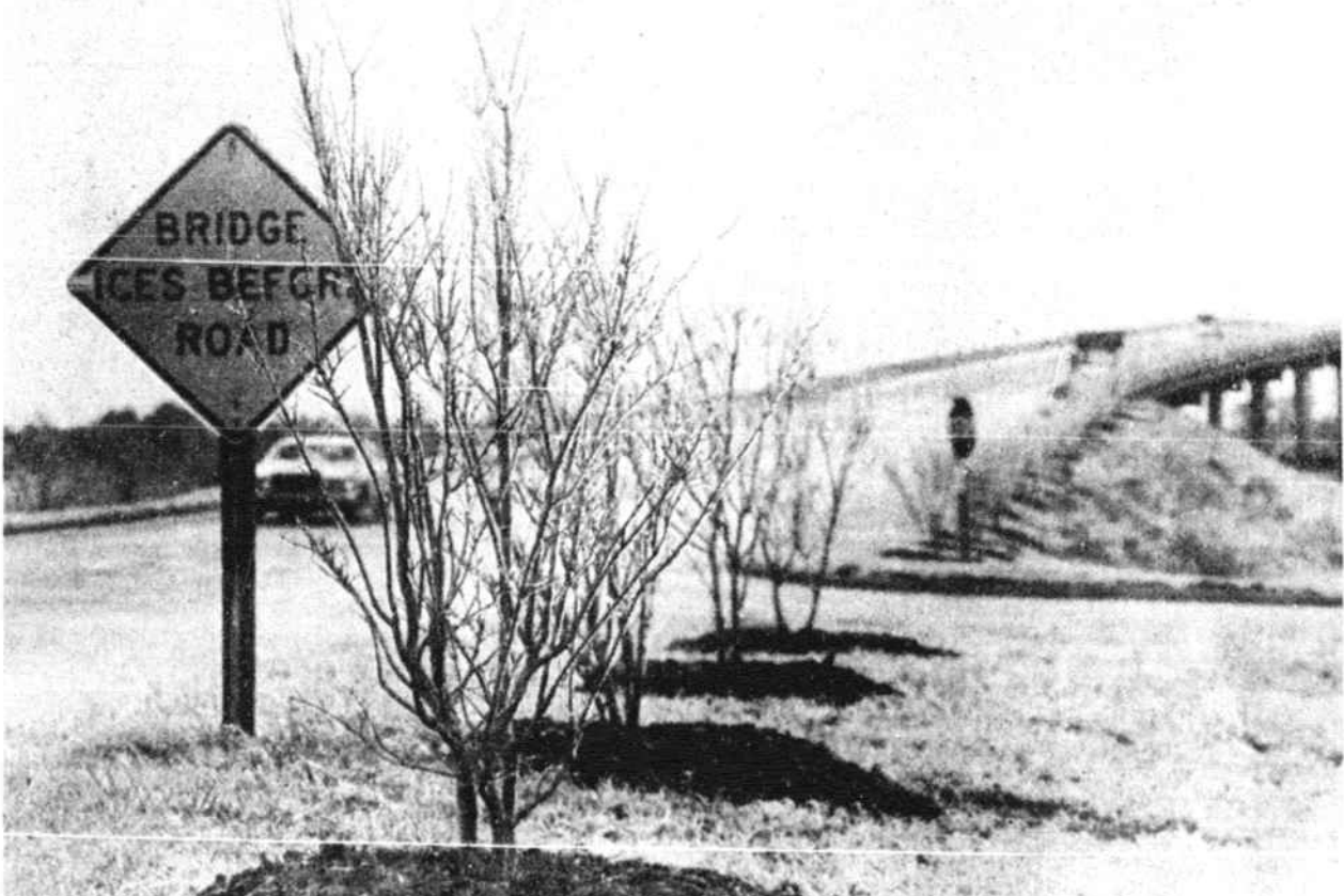
A QUARTER INCH OF ICE coats the limbs of saplings near the foot of the Ocean Isle Beach high-rise bridge Tuesday morning. Despite icy conditions, bridges in the South Brunswick Islands remained passable.
