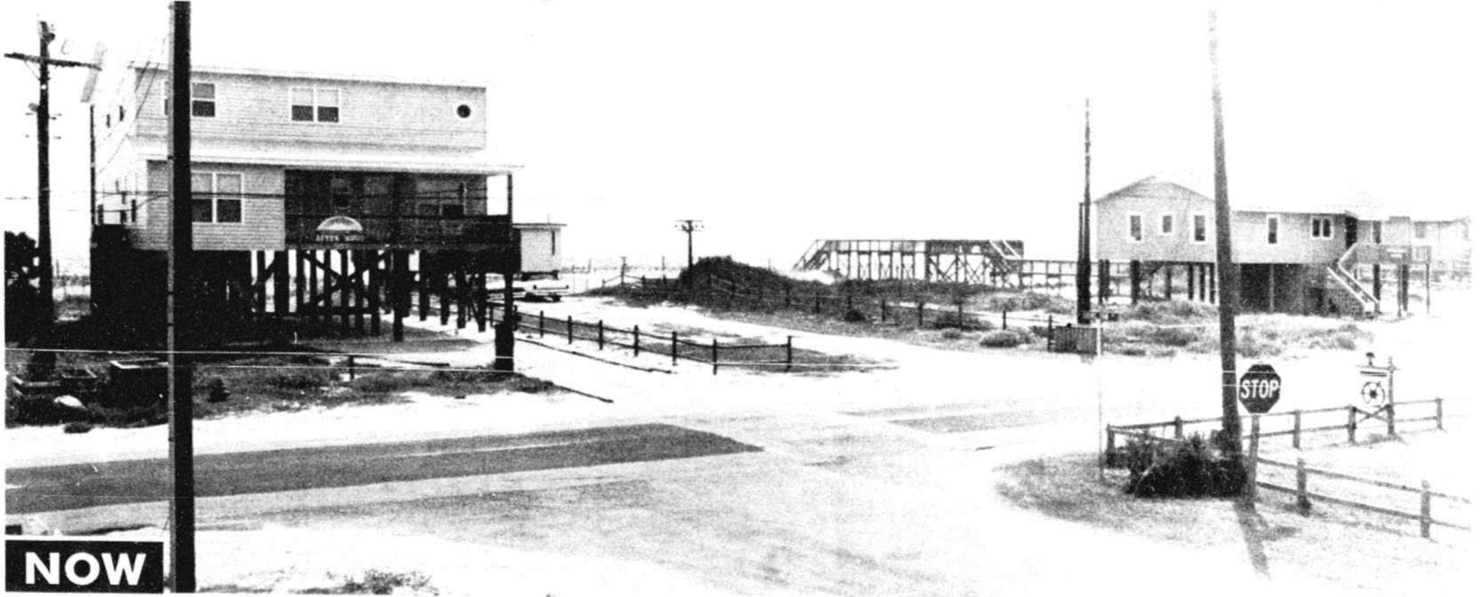
THESE THEN AND NOW PHOTOGRAPHS show the changes that have occurred in the 600 block of Ocean Boulevard West at Lions Paw Drive at Holden Beach since Hurricane Hugo made landfall near Charleston, S.C., last September. The house at right, which was on the verge of collapsing after the storm, has been
