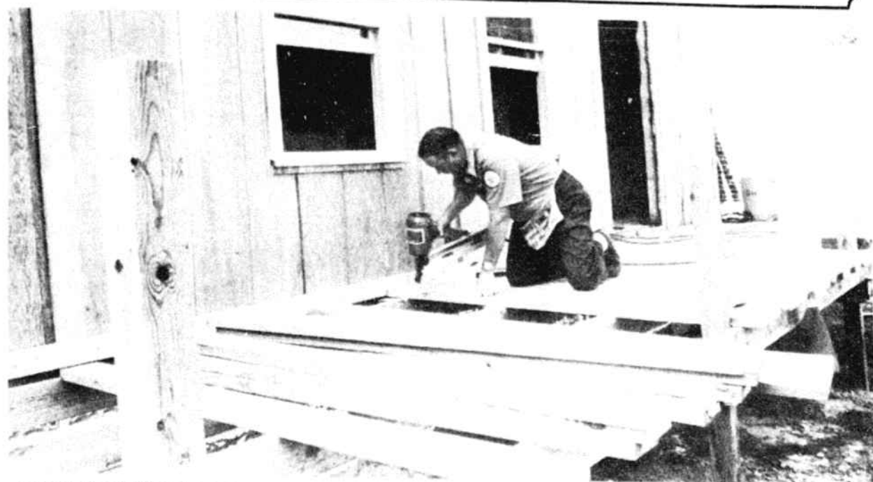
BILLY ROBINSON builds a deck for new office space at the Brunswick County Sheriff's Department.
