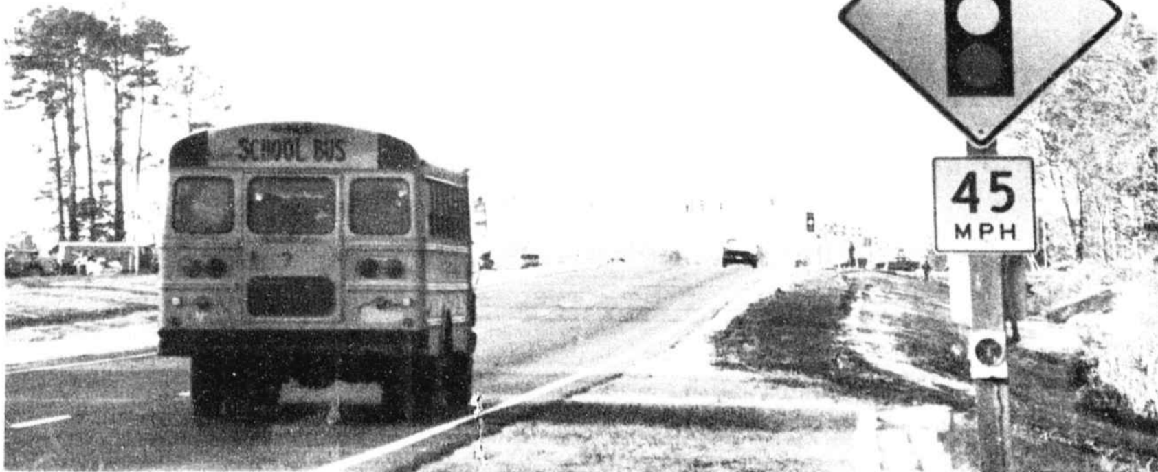
THE N.C. DEPARTMENT OF TRANSPORTATION installed this oversized "signal ahead" sign with a 45 mph "advisory speed plate" and flashing yellow beacon on the U.S. 17 Shallotte Bypass Monday north of the N.C. 130 West intersection.
