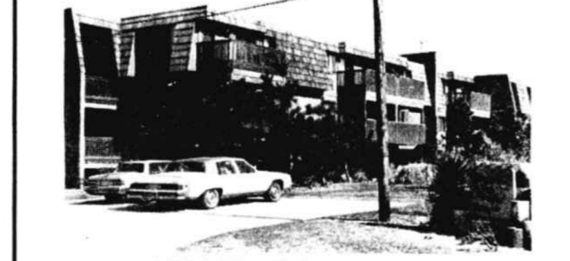
A PLACE AT THE BEACH Oceanfront, 2 BR, 1½ baths, living room, kitchen, air conditioning units in living room and master bedroom, carpeted, dishwasher, furnished, pool. Units available from $59,900.
