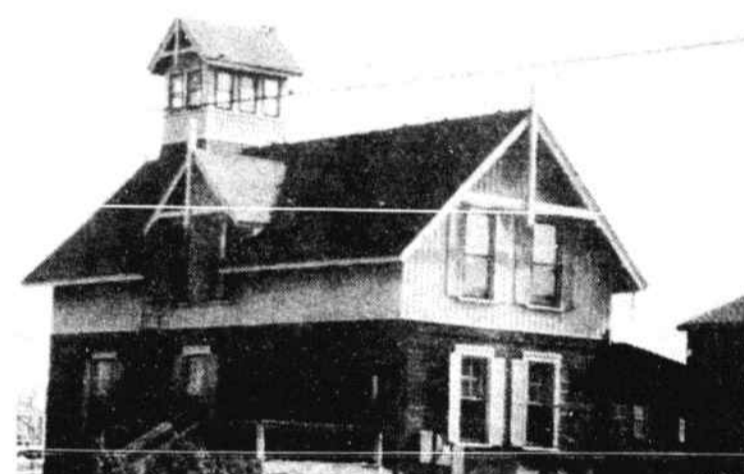
PHOTO BY PATTY JONES PREDECESSOR of the 1932 structure, this turn-of-the-century lifesaving station is now a private residence, situated across the road from the station.
