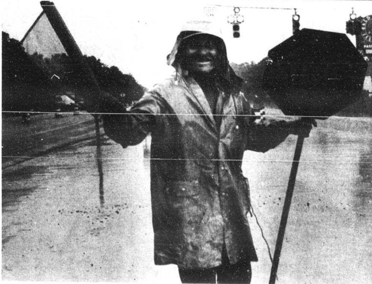
A RAIN-DRENCHED FLAGMAN with Carolina-Dickerson Construction who identified himself only as "Hobo" signals traffic through the busy U.S. 17-Supply intersection during an afternoon storm Monday. Scattered thunderstorms are bringing little relief from the heat and related lightning has caused a series of wildfires across the area.
