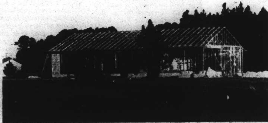
Home under construction near Oriental.
