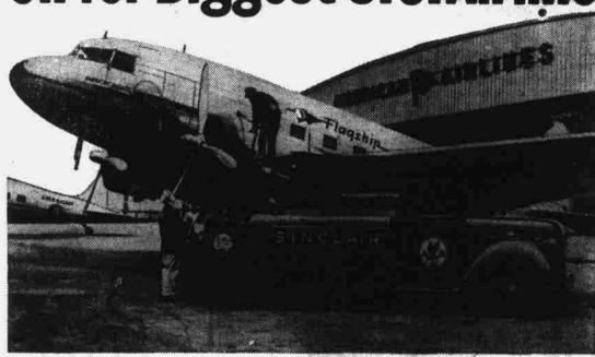
LaGuardia Field, N. Y.-Sinclair's unique oil-jeep drains and fills giant American Airlines' Flagship with Sinclair Pennsylvania Motor Oil. American Airlines, Inc., biggest U. S. Airline, relies on Sinclair Pennsylvania Motor Oil exclusively to save wear on its costly airplane engines.
