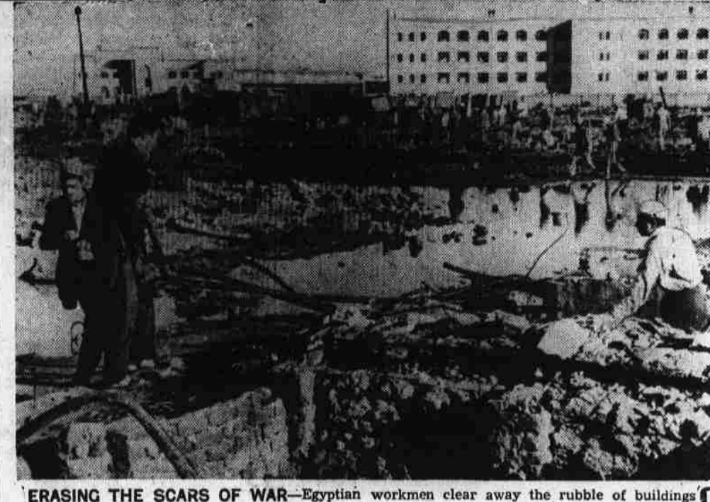
ERASING THE SCARS OF WAR —Egyptian workmen clear away the rubble of buildings smashed by the air and sea bombardment which accompanied the Anglo-French invasion of Port Said. The United Nations salvage fleet has resumed efforts to clear the blocked Suez Canal, of which Port Said is the northern terminus.
