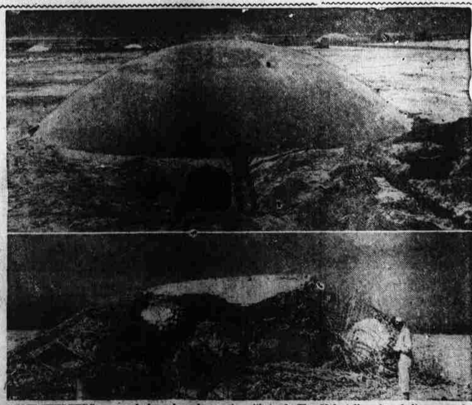
DOMES SHELTERS, a new design whose low cost and easy construction would adapt it to mass production, were tested at the Operation Plumbbob atomic tests in Nevada at pressures from 20 to 70 times those which a house is normally built to withstand. The 50-foot-diameter shelters may be seen before the blast in the upper photo. The lower photo shows one of the domes which was deliberately tested at a pressure so great that it would fail, so its weaker points could be studied. (NTO Lookout Mountain Lab Photo)
