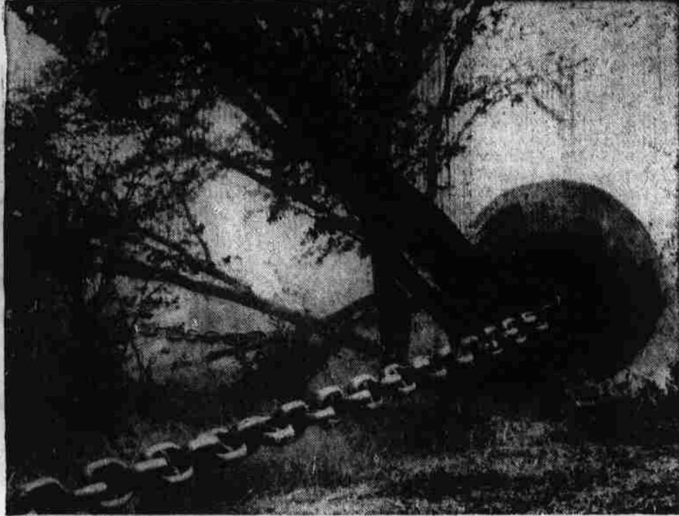
WHAM!—Steel ball at right, some eight feet in diameter, is one of several linked with anchor-type chain to produce a gargantuan land-clearing device at Kariba, Rhodesia. Balls, honey-combed to make them light to tow yet sturdy enough to provide momentum, act as "wheels" for the giant chain. The 100,000 acres being cleared will provide fishing grounds and harbor areas when land behind a new dam is flooded.
