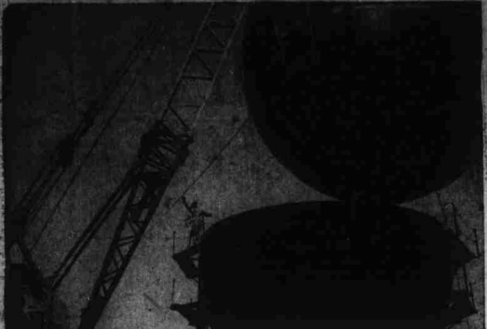
PASS IT TO ME! —Like a basketball player awaiting a rebound in a dream sequence, a worker guides a massive aluminum sphere into place. The metal ball will store liquid hydrogen in Sacramento, Calif.
