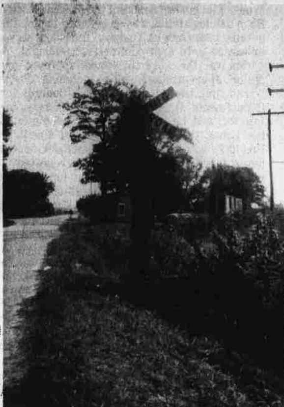
DANGEROUS SIGNAL — This railroad crossing signal in the town of Winfall may be lovely with the rambling vine but it is dangerous for strangers driving through the area.
