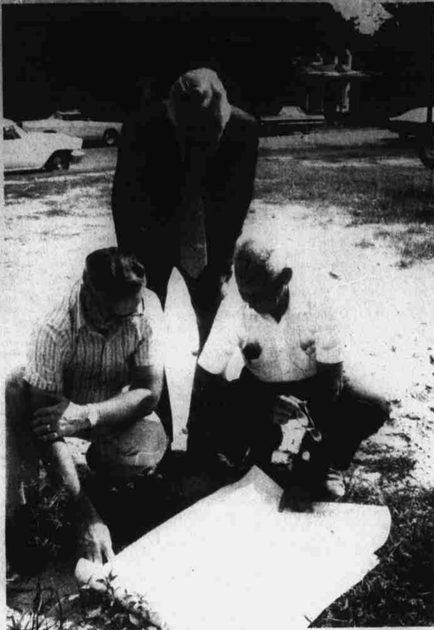
PROGRESS NOTED —Doug Gardner, of Gardner Contractors and Associates (standing) were in Hertford last week with plans and blueprints, making plans and progress on the courthouse annex. The annex will be built where the old jail, which was torn down recently once stood. (Sawyer Photo)
