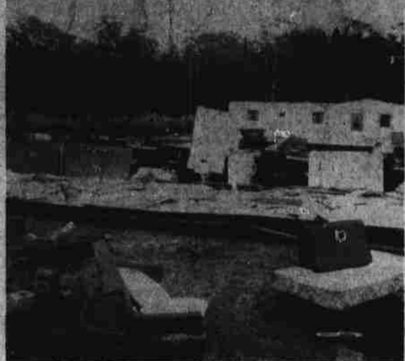
TORNADO DAMAGE —A tornado which swept through the Holiday Island community of Perquimans County left this mobile home belonging to Martin F. Bremus in total
