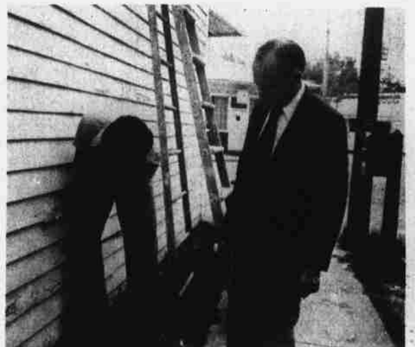
NEW LOOK — Keith Haskett's grocery store, on the corner of Market Street, has been sold to the S & R firm in Elizabeth City. Max Mercer, general manager of the stores, supervises some outside renovation of the store. The deal was closed Monday.
