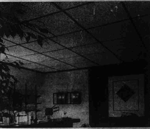
These handsome 2' x 2' panels, with heavy stucco texturing, create a dramatic shadow effect because the black contrasting grid is recessed. The sound-absorbing fire-retardant panels install quickly and easily without special tools . . . we'll show you how!
