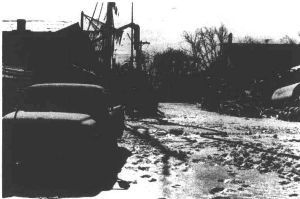
ERIE — Shadows and a combination of fighting present an eerie looking scene at the fire site Wednesday morning.
