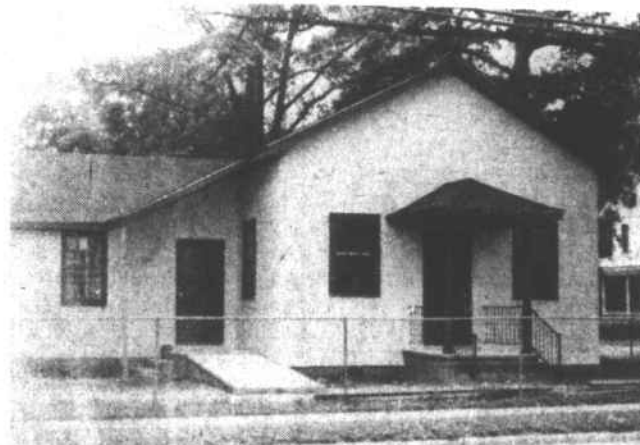
NEW CENTER — This is the new Senior Citizens Center on Grubb St., across from the Parks and Recreation Department office. Work on the exterior has been completed and the interior should be completed by mid-August according to Billy Wooten, Parks and Recreation Department director. (Staff photo by JACK GROVE)
