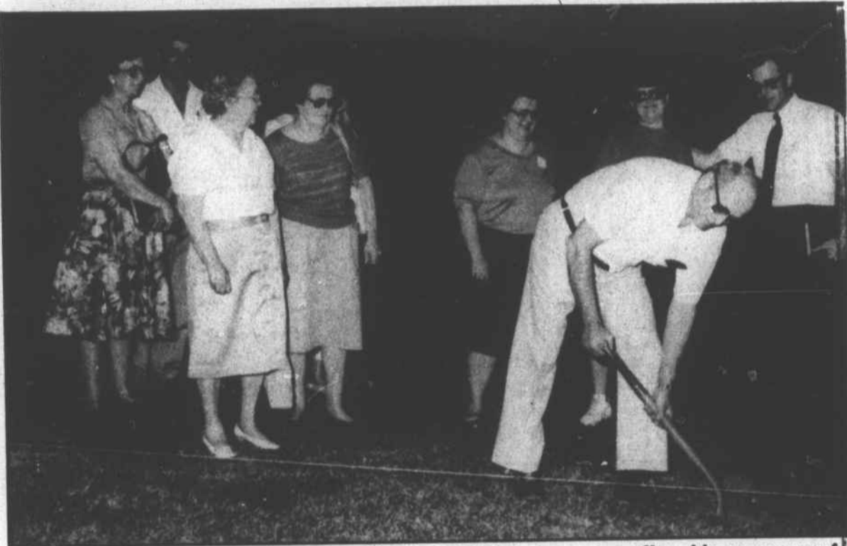
GROUNDBREAKING —John Mansfield, Chairman of the Board of Deacons at Mt. Sinai Baptist Church recently turned the first shovel of dirt during a groundbreaking ceremony for the church's new fellowship building.
